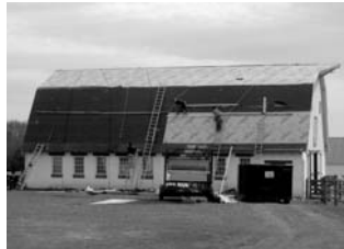
A new roof for the pig barn
